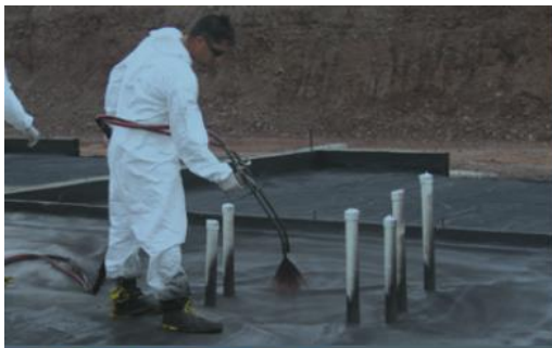
Figure 11. Spraying an emulsified asphalt latex barrier.
